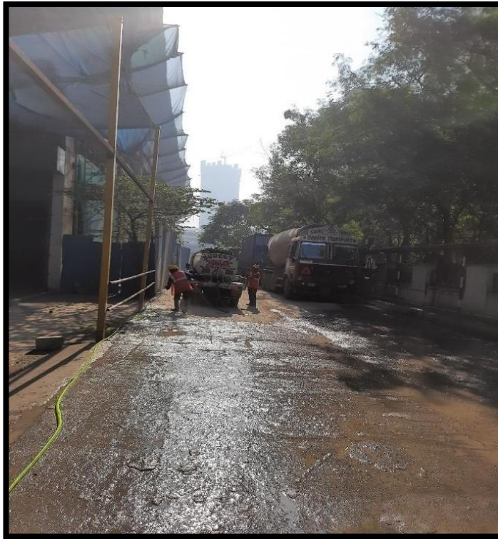
ACCESS ROAD IN THE SITE
