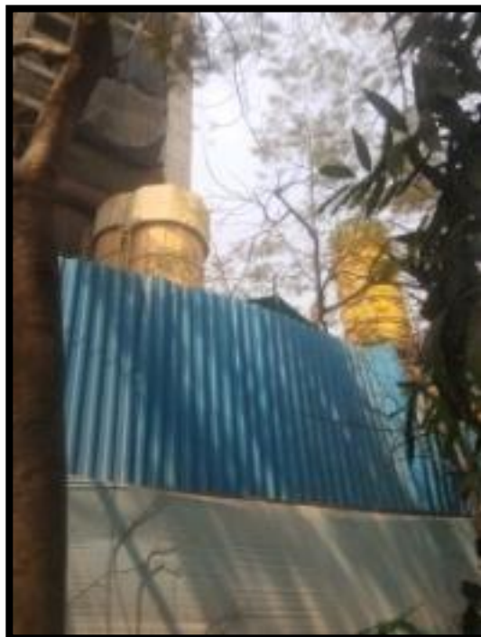
METAL BARRICADING FOR NOISE ABATEMENT
