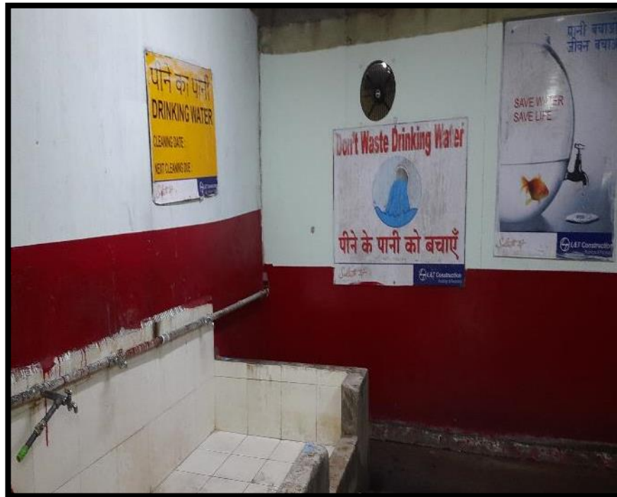
WATER SUPPLY WORKERS ON SITE
